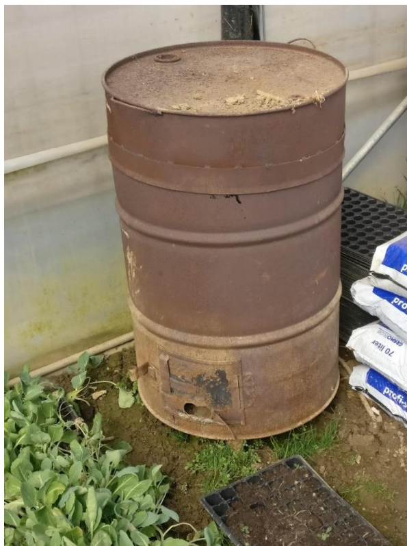
Figure 7: Drum stove heating system to heat tunnel for seedling production shown at left. Insulation for lower portion of tunnel walls shown at right.
